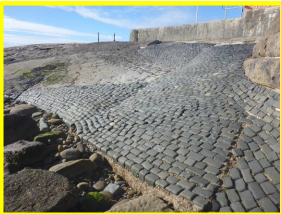
Tie-in section between wall and pier (/4701C06)
