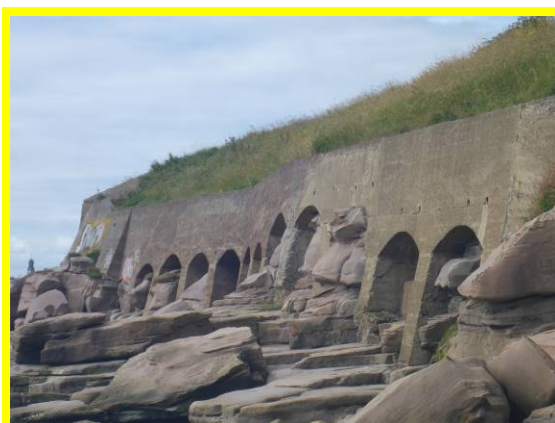
Masonry and concrete arched seawall (/4801C04)
