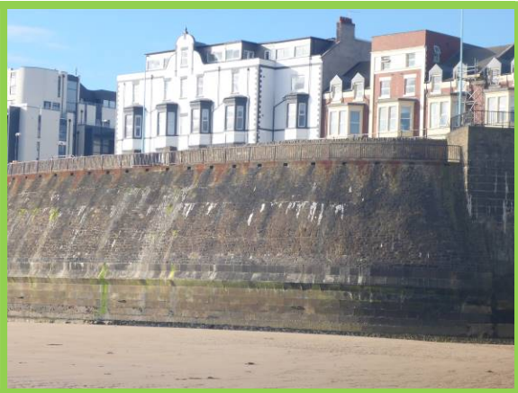
High blockwork sea wall (/4601C05)
