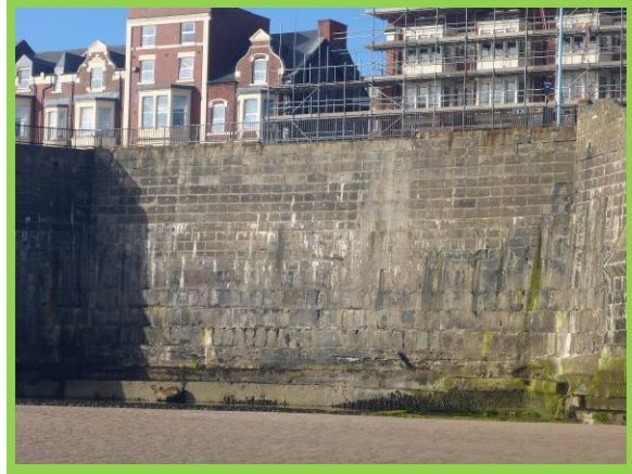
High blockwork sea wall (/4601C04)
