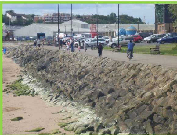
Masonry and concrete arched seawall (/4801C09)
