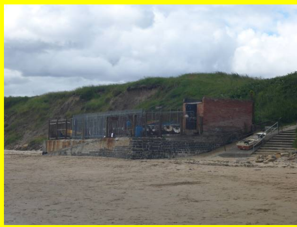
Wall at boatyard (/4501C05)
