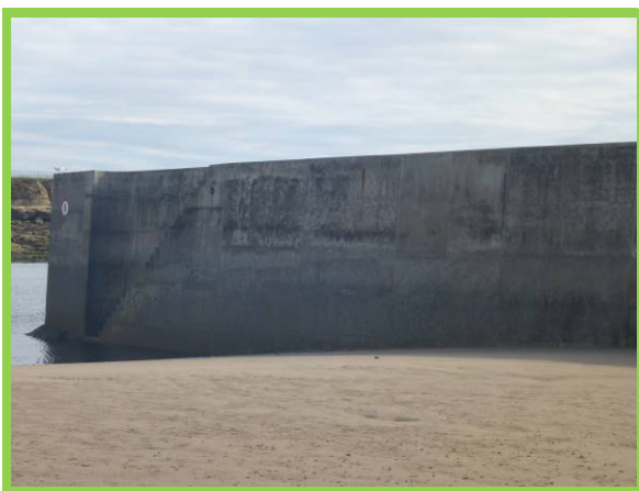
Cullercoates South Pier – deck and vertical landward face (/4701C15)
