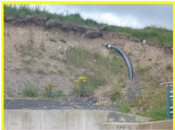
Drainage added to cliffs above the T-Blocks (/4501C05)
