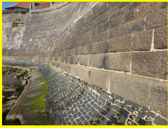
Final section of sea wall in generally fair condition (/4701C06)
