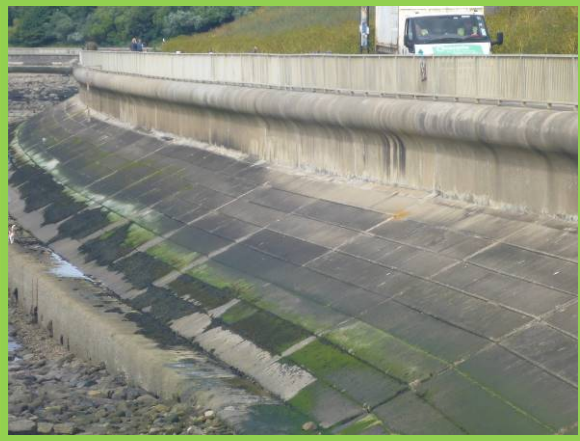
Concrete panel sloping revetment and short concrete toe wall (/4801C07)
