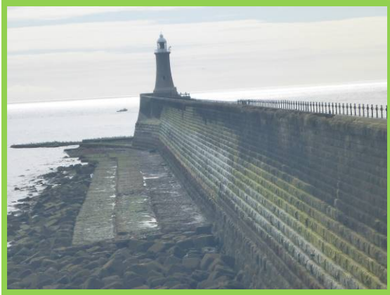
North Pier appears in good overall condition and is well maintained (/4801C01)
