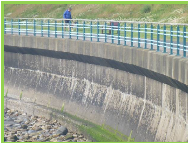
Trinity Road seawall in good overall condition, but with some minor maintenance required (/4501C04)
