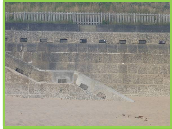
Seawall and access ramp (/4501C07)
