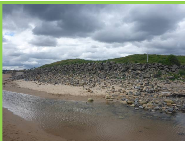
Rock revetment near Briardene Burn (/4501C06)
