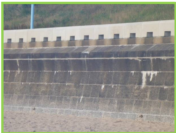
New coping on blockwork seawall (/4501C07)
