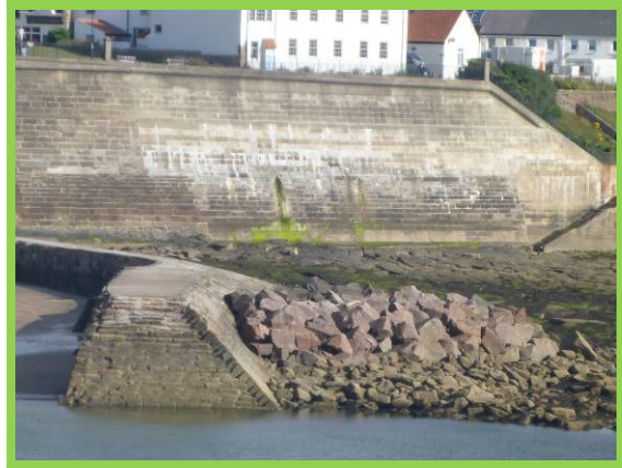
Cullercoates North Pier – seaward end with rock armour emergency repair (/4701C07)
