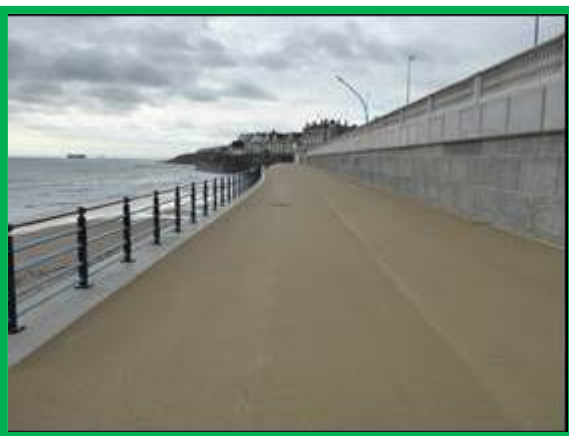
Refurbished promenade (/4601C03)
