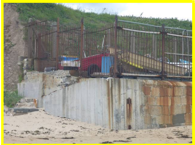
Wall at boatyard (/4501C05)
