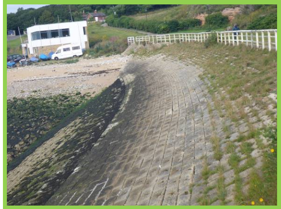
Masonry revetment (/4801C02)
