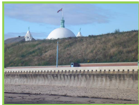
New coping on concrete recurved seawall (/4501C08)
