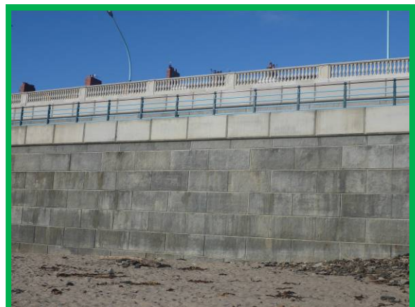
Refurbished sea wall (/4601C03)
