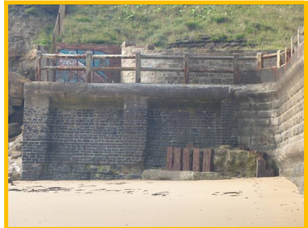
Tie-in wall between Outdoor Pool and undefended rock cliffs (/4701C25)
