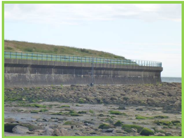
Trinity Road seawall in good overall condition (/4501C04)
