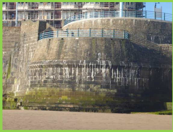
Blockwork sea wall at first 'bullnose' (/4601C04)
