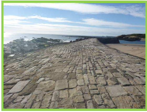
Cullercoats North Pier – sloping seaward face (/4701C07)
