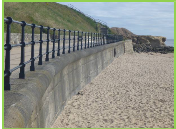
Higher beach levels at wall's toe in 2020 inspections (/4701C18)
