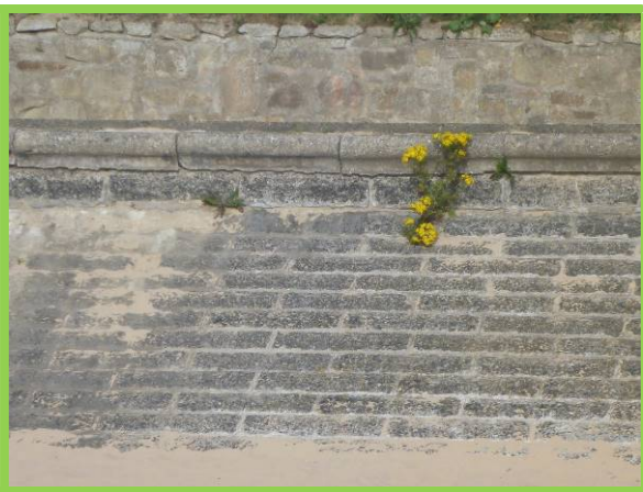
Sloping blockwork revetment (/4701C19)
