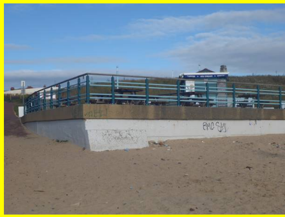
Refurbished seawall north of beach access ramp (/4501C09)
