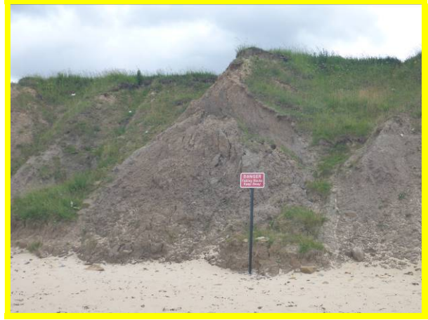
Recently erected warning signs (/4501C05)
